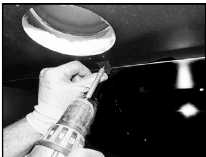
Figure 11.5 Install Back Glass Panel Retaining Bracket
